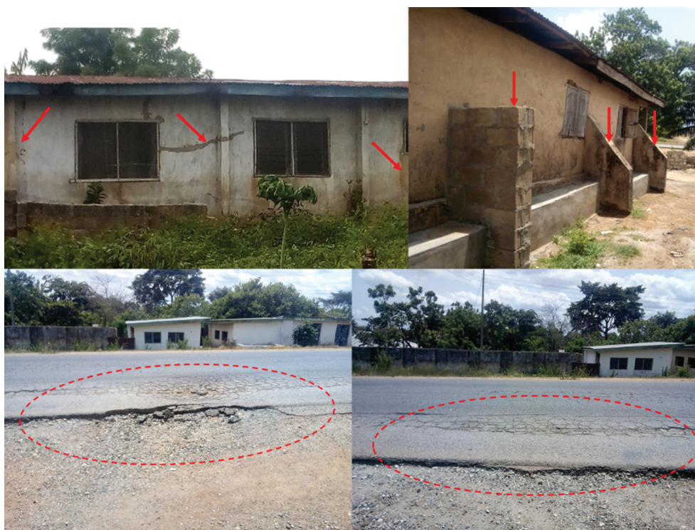
Figure 1. Images showing some of the defected engineering structures in the study area. The red arrows indicate reinforcements (concrete patching and buttress supports), while the red circles show the sections of the highway with pavement defects.
