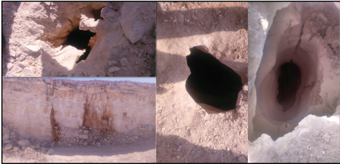
Figure 1. Examples of founded caverns that were uncovered on the construction site during excavation.
